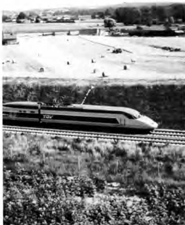
Depending on terrain, the strip of land required for the VFT may be as narrow as 40 metres in width. Agriculture can proceed undisturbed alongside the railway alignment, as shown in the picture of a TGV in France. —photo SNCF
